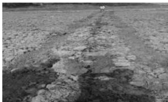
Plate 2.5 a Digging of Main drain for laying mole drains (The shallow water table resulted in seepage into the main drain). Preparation of pipe bends for mole drains
