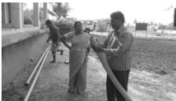
Plate 2.5 a Digging of Main drain for laying mole drains (The shallow water table resulted in seepage into the main drain). Preparation of pipe bends for mole drains
