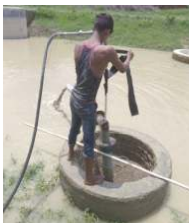
Cleaning of recharge well by compressor
