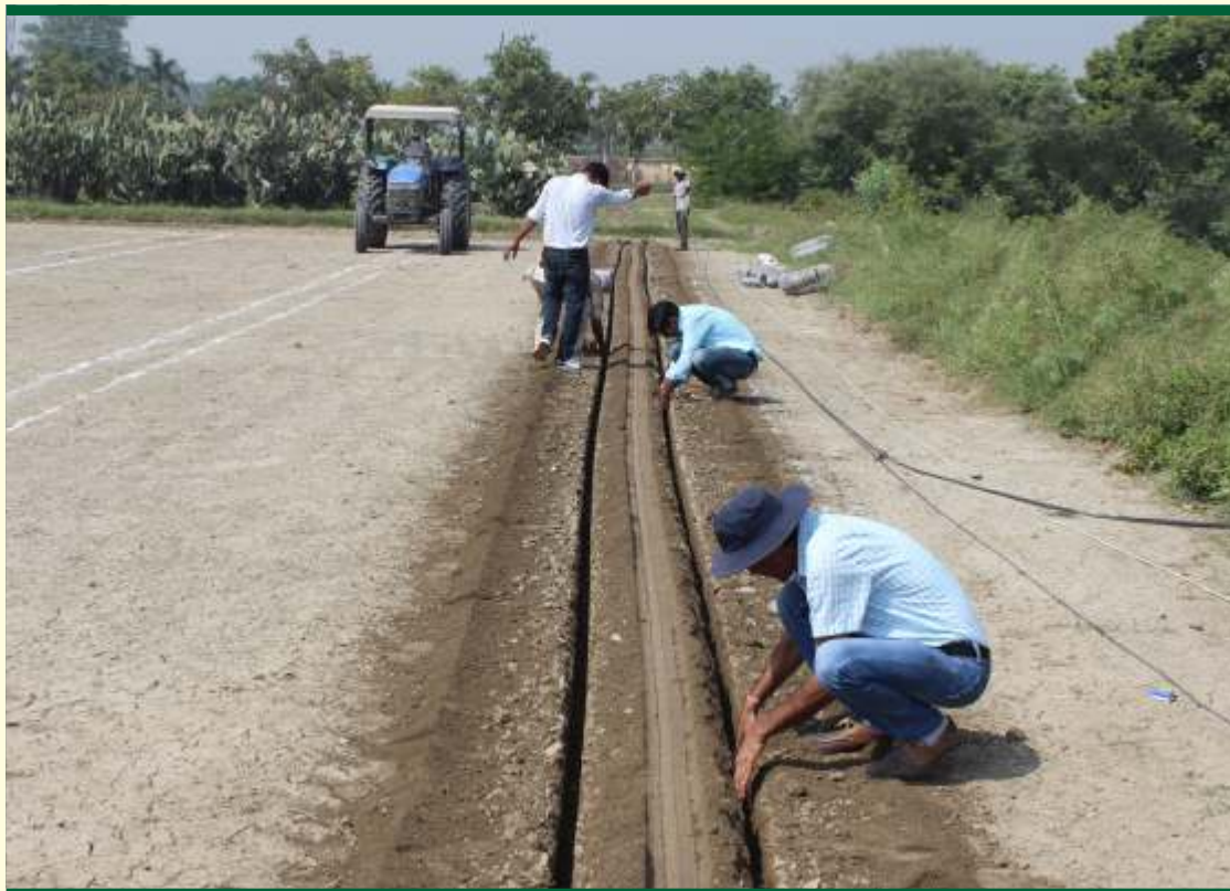
Plate-6 Drip lines installation in trenches
