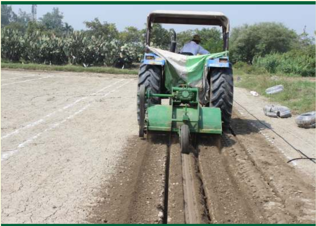
Plate-5 Digging of trenches with a tractor-drawn drip-trencher in moist soil
