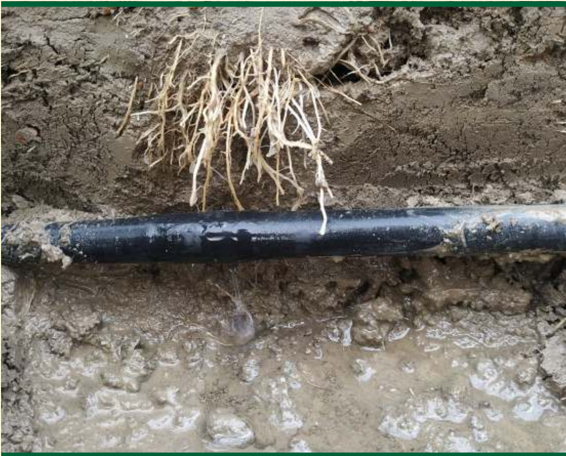
Plate-7 Irrigation through subsurface drip in crop root zone
