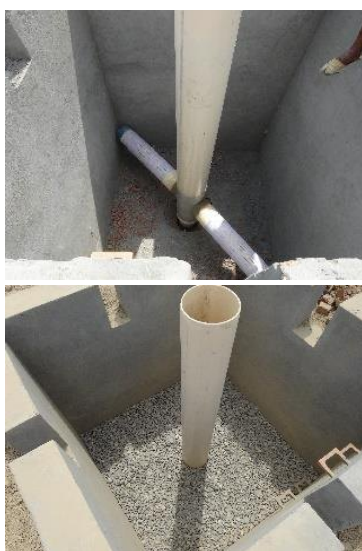
View of recharge arm at the bottom of filter chamber and covered with boulder
