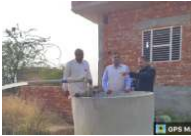
Pumping of drainage water from a SSD block into Kahni open drain
