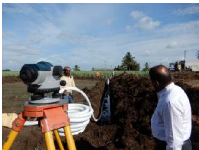
Installation of SSD system, transformed barren field into lush green cane field at Majrewadi (Kolhapur)
