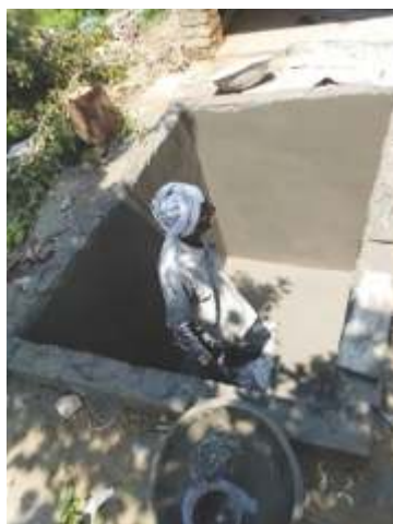
Construction of rain water storage tanks.
