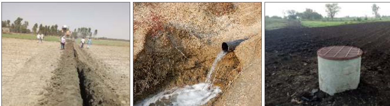
Semi-mechanical installation of SSD work with Hydraulic excavator in Arjunwad (Kolhapur) and manhole installed in the field
