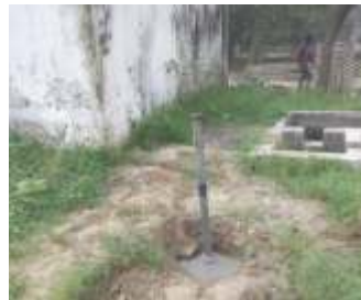
Installation of observation well
