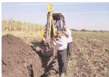
Mechanical excavation of trenches
