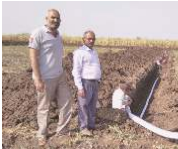
Manual laying of SSD pipes
