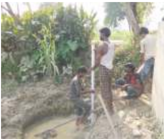
Installation of observation well
