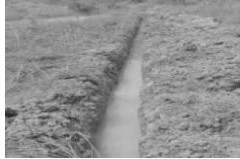
Plate 2.5 a Digging of Main drain for laying mole drains (The shallow water table resulted in seepage into the main drain). Preparation of pipe bends for mole drains
