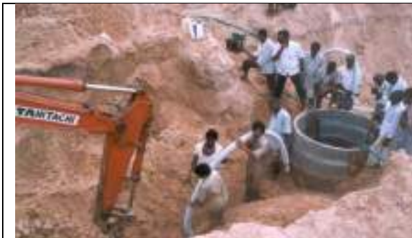
Construction of new Doruvu technique
