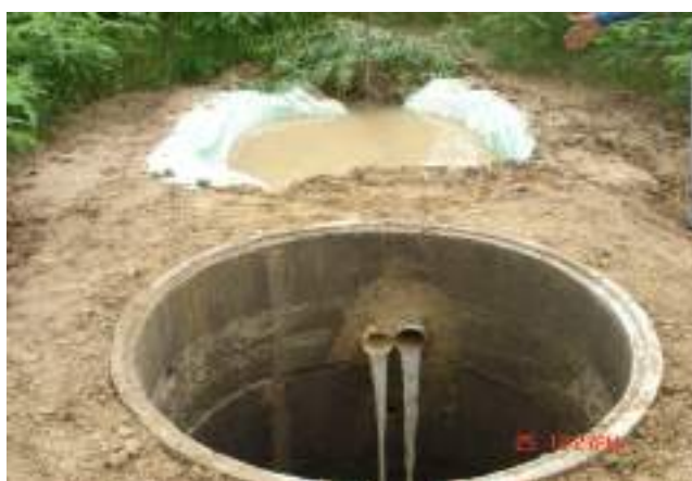
Fig. 50 Rainwater recharge to dilute groundwater
